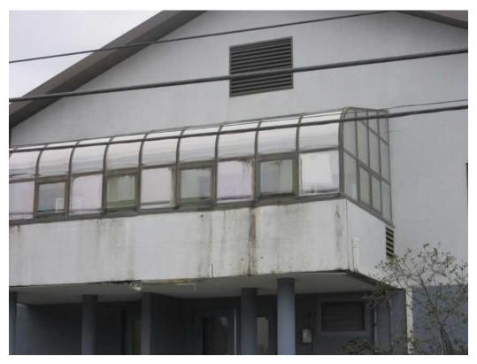
Figure 2-5: Cladding Damage at Long Term Care Wing Exterior Sun Room
